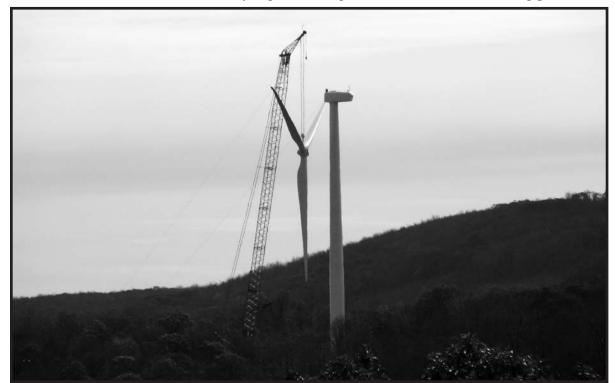
A CRANE LIFTS blades to be mounted to a turbine at the Beech Ridge Wind project in Greenbrier County. Almost 200 local union construction workers got to work on the Beech Ridge project before it was shut down by a Federal Judge from Maryland because of claims made that the endangered Indiana Bat was being affected.
